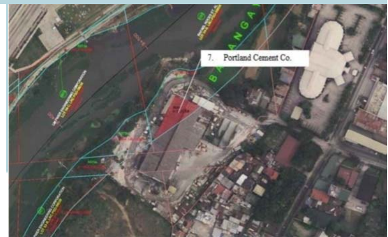
Affected industrial lots with structures
